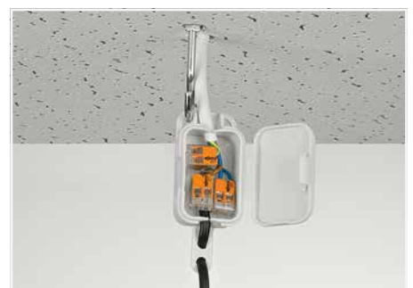
Pendant light connection in suspended ceilings
