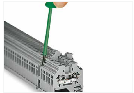
Removing a terminal block from the assembly.
