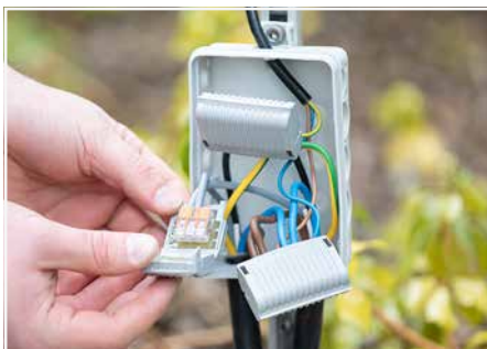
Connecting a bollard light
