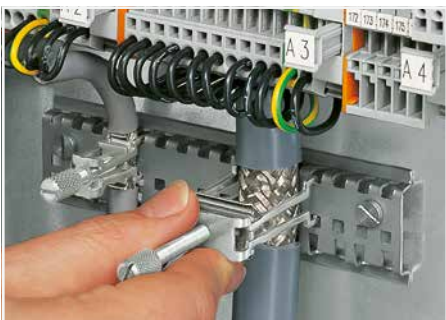
Securing an additional shield clamping saddle.
