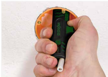
Stripping a cable sheath.
