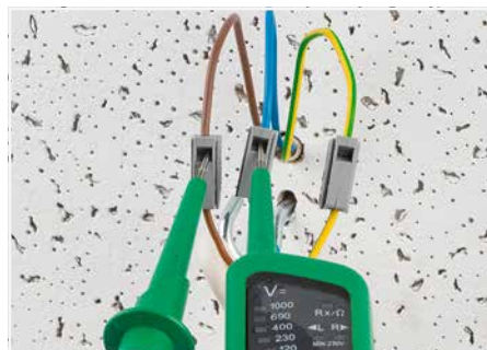
Testing via separate test ports.
