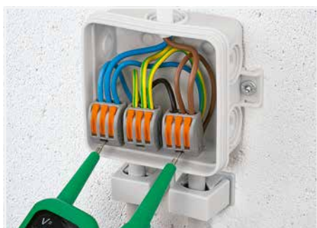
Testing the wired connectors.
