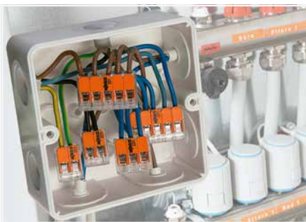
Wiring fine-stranded conductors in a junction box for in-floor heating.
