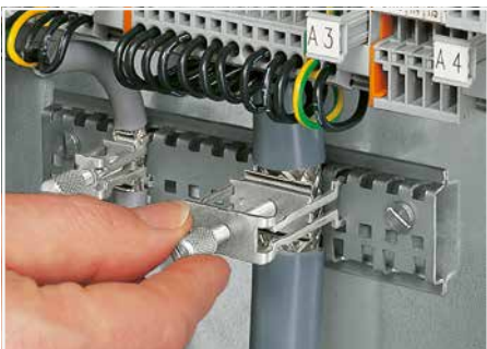
Tightening/removing a shield clamping saddle.
