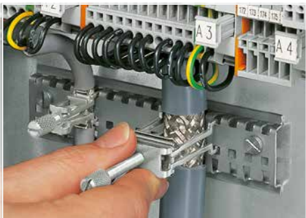
Securing an additional shield clamping saddle.
