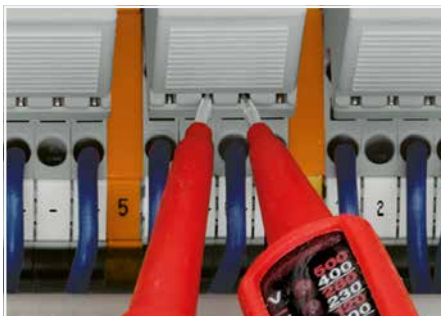
Function testing via touch-proof test slots.
