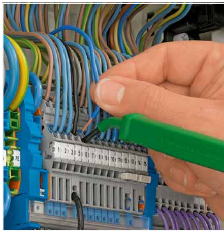
Open the clamping unit using an operating tool.
