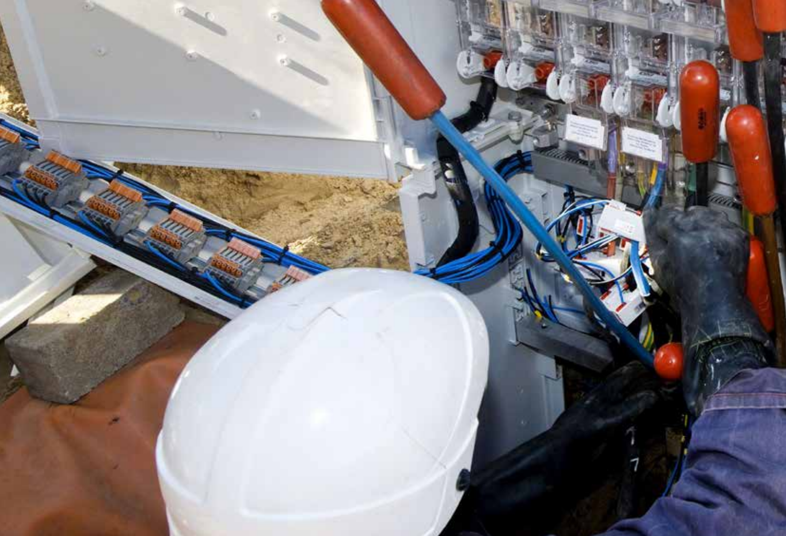
Upgrading the electrical system up to the distribution box
