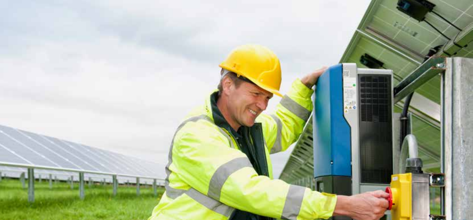
Solar engineer connecting an inverter
