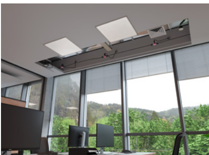
Installation of shading systems
