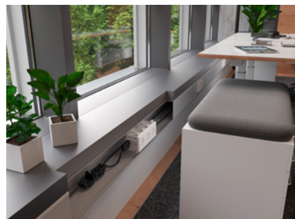
Installation of cable duct systems
