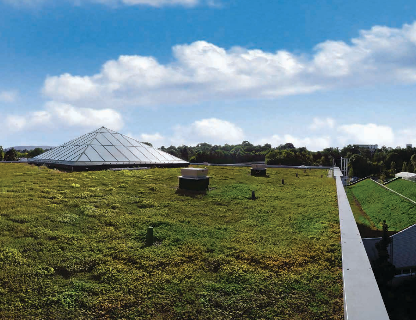
Green WAGO roofs
