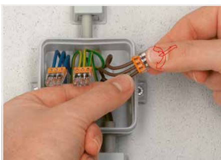
Removal: Hold conductor to be removed and twist alternately left and right while pulling the connector.
