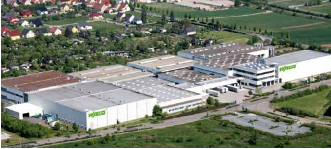
WAGO Sondershausen, Germany
