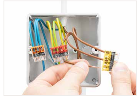
Termination: Insert the stripped conductor until it hits the backstop.
