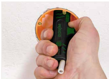
Stripping a cable sheath.
