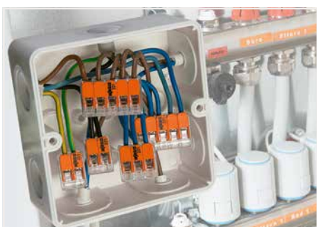
Wiring fine-stranded conductors in a junction box
